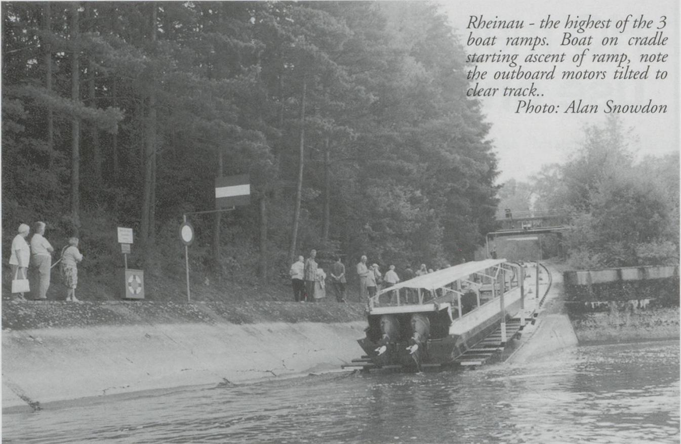
*Rheinau - the highest of the 3 boat ramps. Boat on cradle starting ascent of ramp, note the outboard motors tilted to clear track..*
