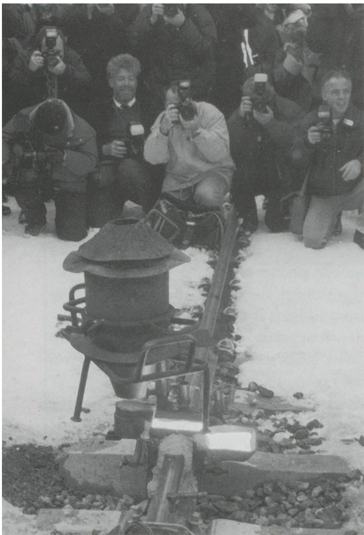
Molten metal flows through to join the rails as the worlds railway press snap in unison.
