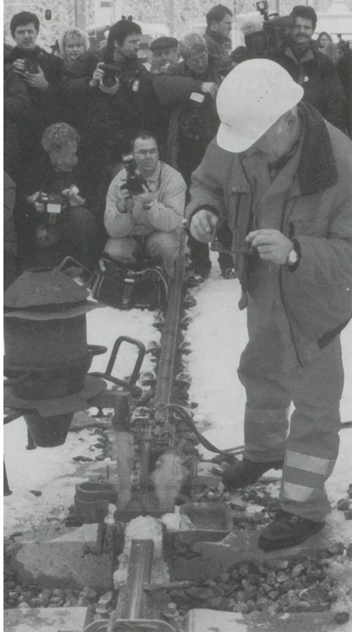
*The RhB's Chief Engineer, Willy Altermatt prepares the thermic weld at Selfranga joining the rails.
