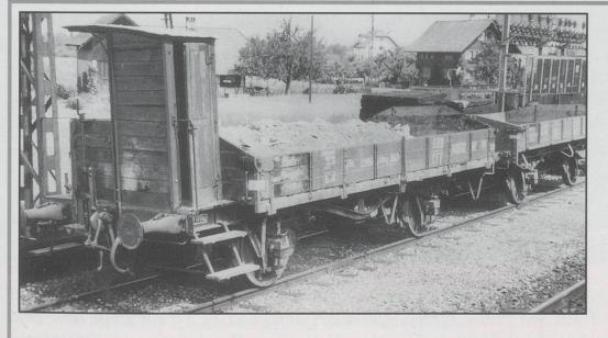
This open wagon dates from 1891 and was 62 years old when it was photographed at Brügg. A feature of the wagon is the semi-open brakesman's cabin. scant space available and
