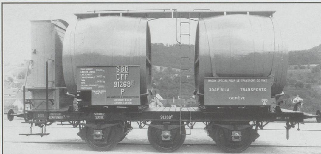
3-axle wagons were in a minority amongst the Swiss wine wagon fleet, numbering about 40 in a total of 960 in 1924. This example, P 91269, was operated by the Geneva Company "José Vila". As well as being renumbered in 1924 to P 521354, it passed through several other ownerships before being withdrawn in 1950. Livery is uncertain, but was probably grey, with the principal lettering in white, shaded black. The centre wheelset seems to have been included purely for weight reasons, as it is unbraked.
