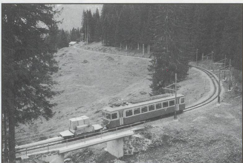
1). The enclosed photograph shows a Grützschalp-bound train of the BLH crossing the new bridge over the Staubbach; the previous bridge having been demolished by an avalanche in February 1999, closing the line for a couple of months I believe. The photo was taken on the 13th September 2001
