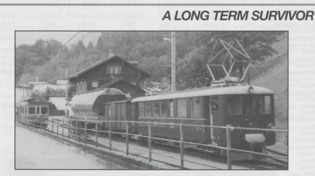
Swiss Express 6/6 carried a picture, under the heading Past Times, of GFM (now TPF) Be4/4 of 1905 vintage. The automotrice is alive and well and on 5/9/01 was working as the station pilot at Broc Fabrique in pouring rain and such poor light that Michael Farr's camera flash worked involuntarily! The regular service was provided by BDe4/4 124 which is waiting in the platform to detach its milk tank.
