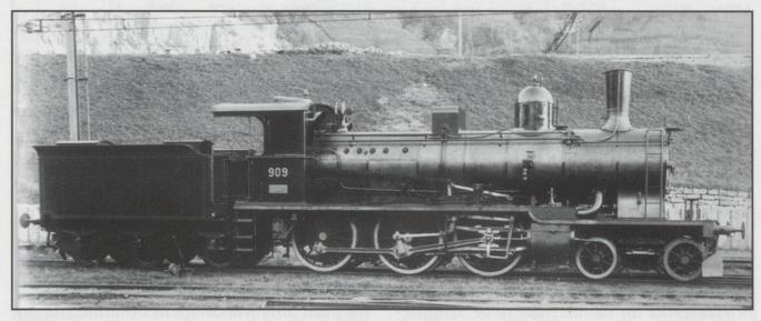
dome. A sand box located above the mid point between driving axles one and two fed sand to the leading edge of both. Adhesion weight of the locomotive was 46 tonnes.
