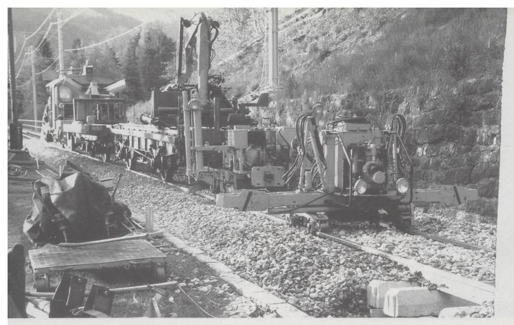
Above: The next strange looking collection of machinery awaits the cranes to move along laying the new sleepers.
