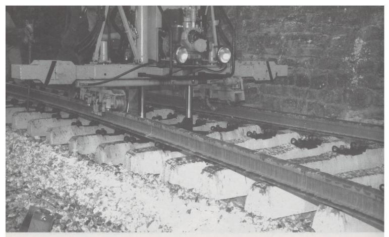
Above: The small machine uses hydraulics to lift the rails onto the metal chairs. Below: The importance of placing the track back in exactly the same position as it came from not only affects the clearance from walls etc. but also where the pantograph connects with the overhead line.
