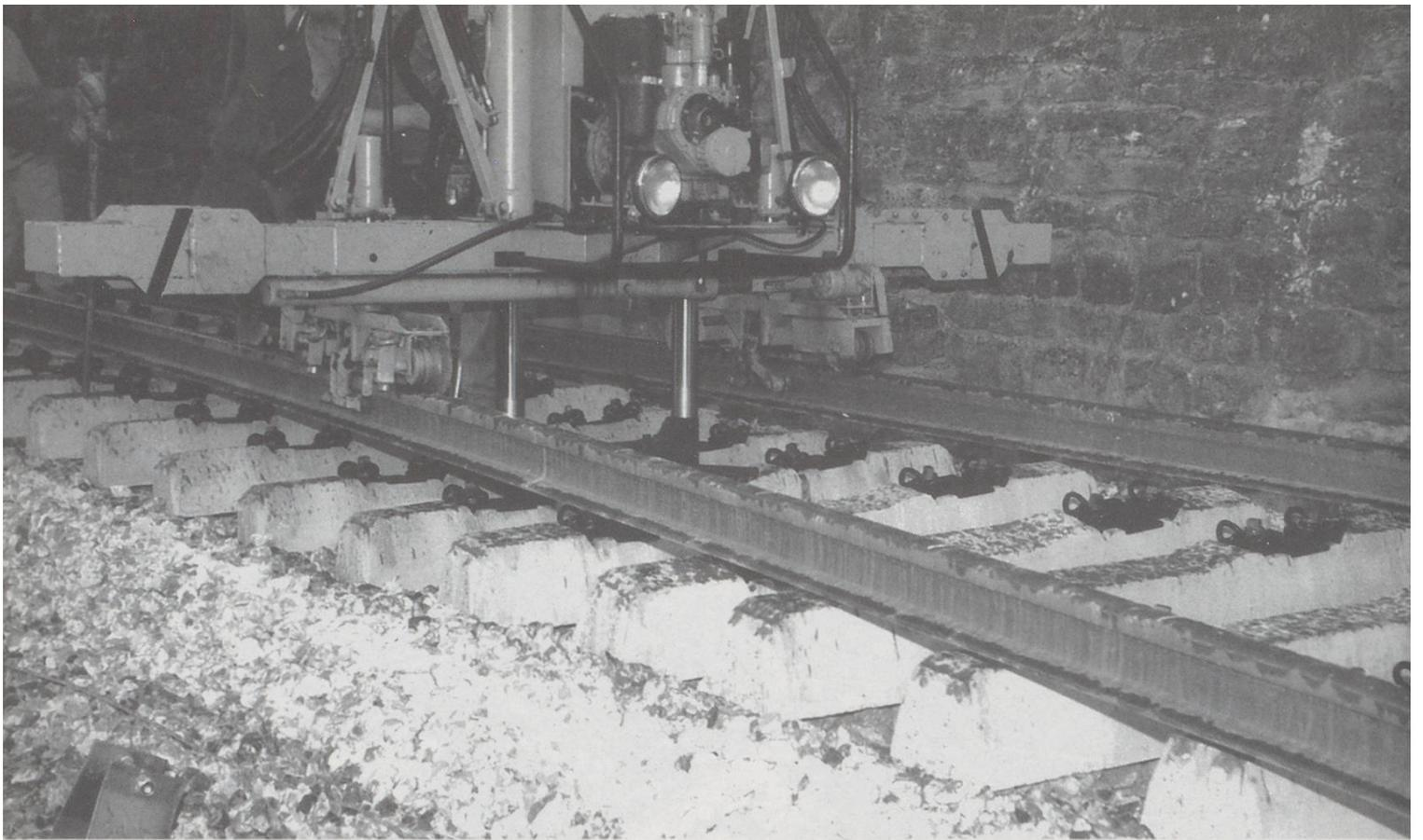
*Above:* The small machine uses hydraulics to lift the rails onto the metal chairs.
