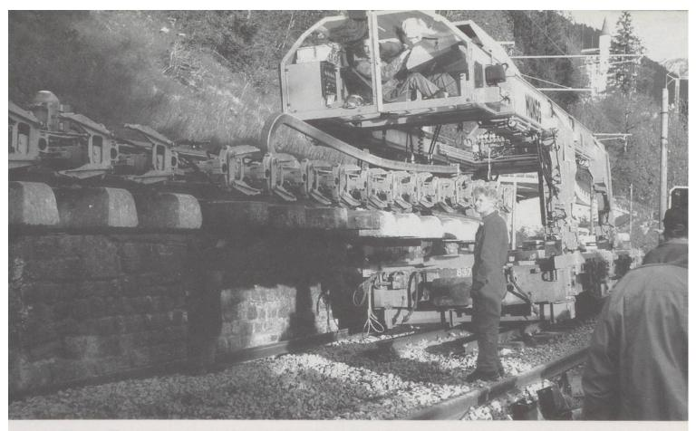
Above: The section of old track being manouvered under the wagon crane, to be carried along the train and placed onto one of the empty flat wagons.
