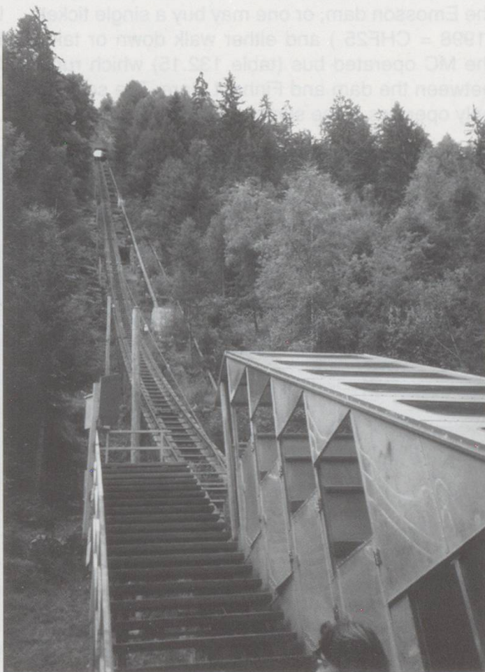
Le Châtelard: Lower Funicular showing the haulage rope lifted well off the guides. Photo: Anne Williams
