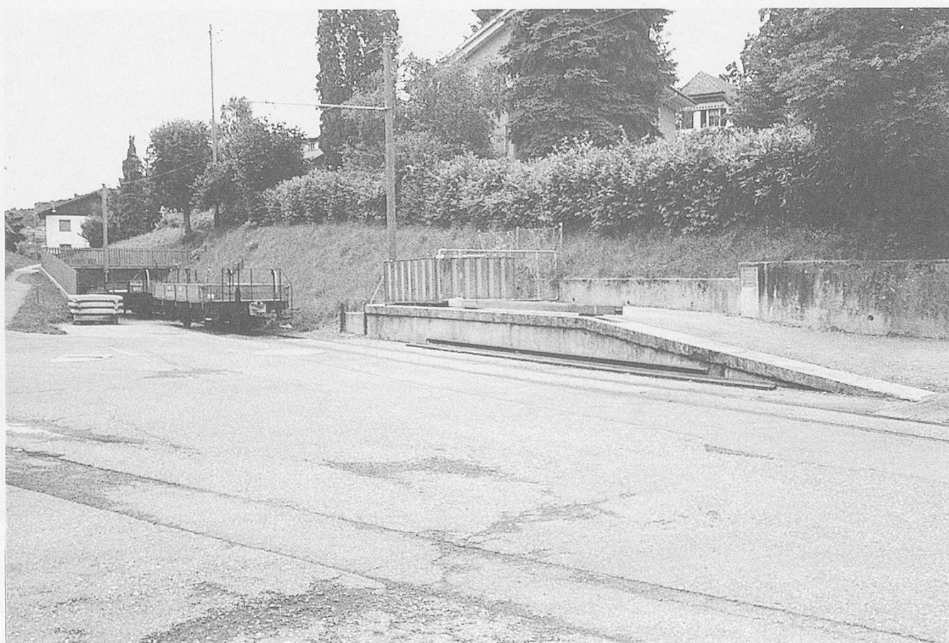
The goods ramp and siding leading into the former cutting. The "track marks" are visible in the foreground
