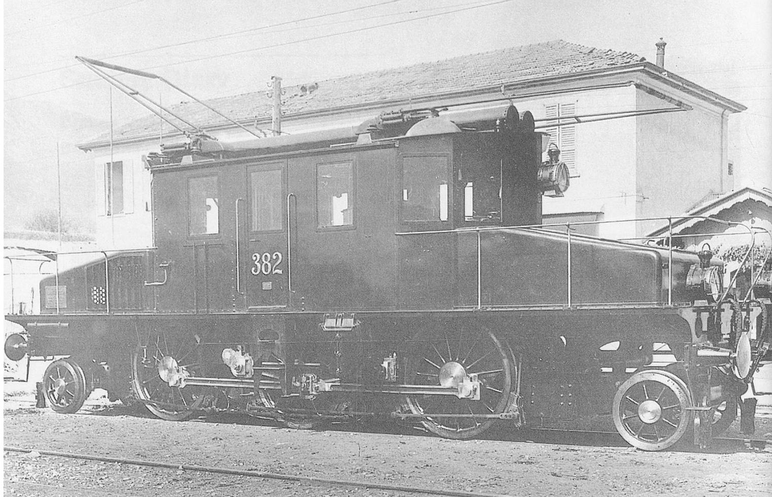
Corresponding to the Simplon N0.362, FS No.382 is of the same type, and shows the simple type of current collector fitted to the Ganz locomotives.
