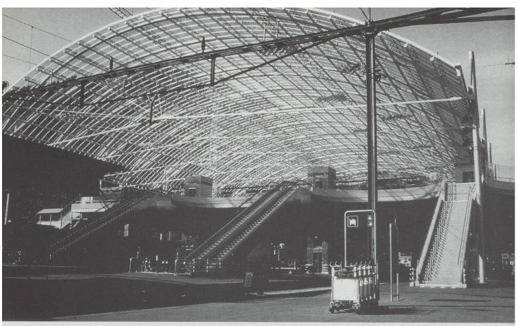
Above: The high level Post bus station that has been constructed over the main station at Chur. Photo G.J.S.Carr Below: The two open coaches obtained from the Brünig line now in service on the Aigle-Sepey-Diableret (ASD)
