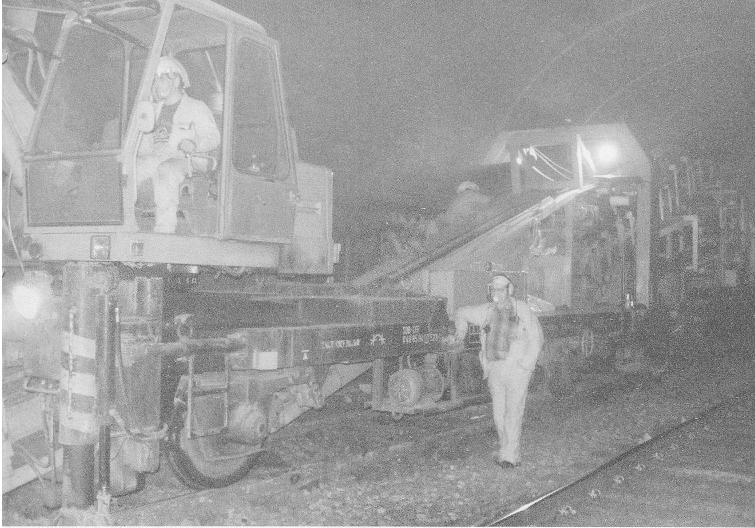
Several solutions were proposed, but since all construction had to be done with the full existing traffic running through at all times, these were rather limited. The final solution involved lowering both tracks 100 mm, as well as moving the right hand track (as seen from Kandersteg) over by 100 mm. This will allow for a *Huckepack* train with 4.0 m corner height lorries running on the left hand track to pass normal outline trains running on the right hand track.
