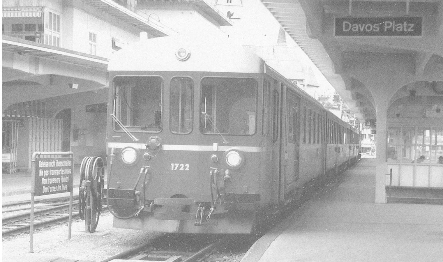
Above: Bdt 1722 heads train 145, the 13.52 to Filisur, at Davos Platz on June 24th 1995. The remodelled cab front with the removed gangway door is clearly visible.
