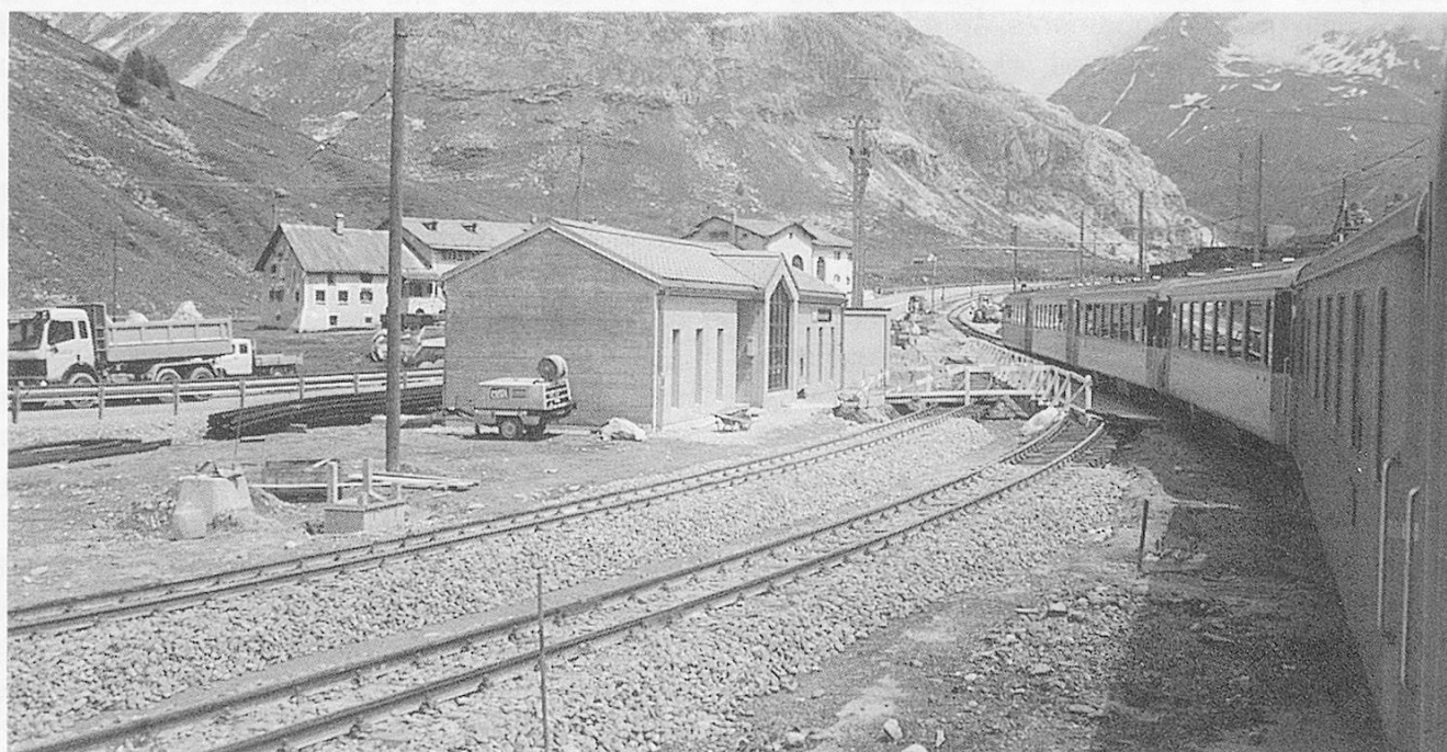
Bernina Suot, 21 June 1993, showing new station building, realigned road and new loop under construction. Photo Nick Freezer.
