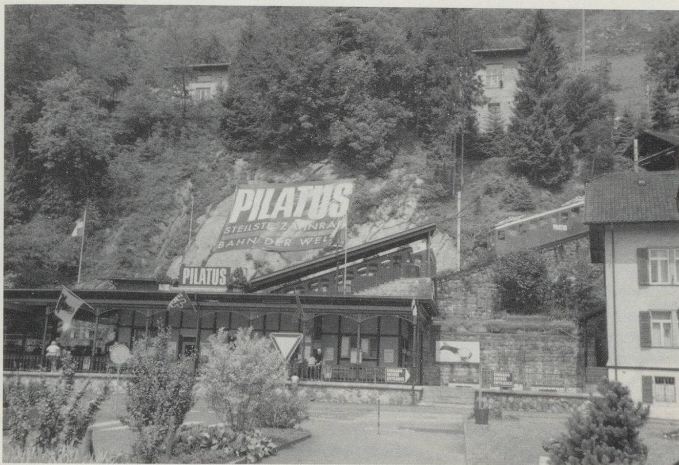
The lower terminus of the Pilatusbahn at Alpnachstad: 16 June 1992
