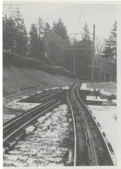
Traverser "points" at Aemsigenalp passing loop.
