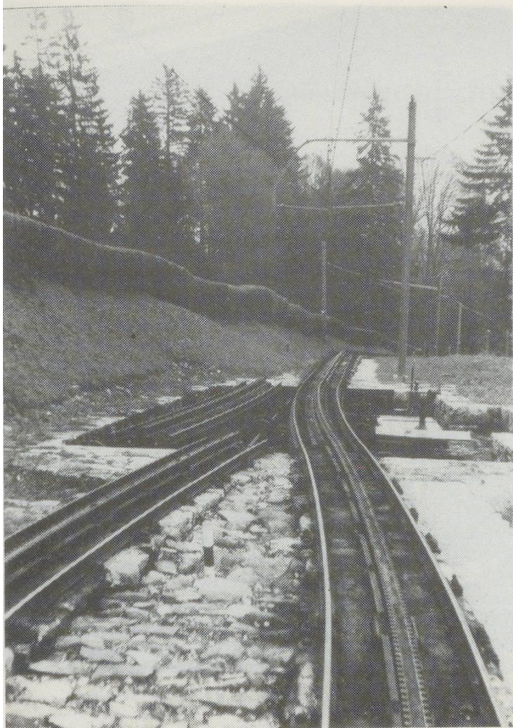
Traverser "points" at Aemsigenalp passing loop.
