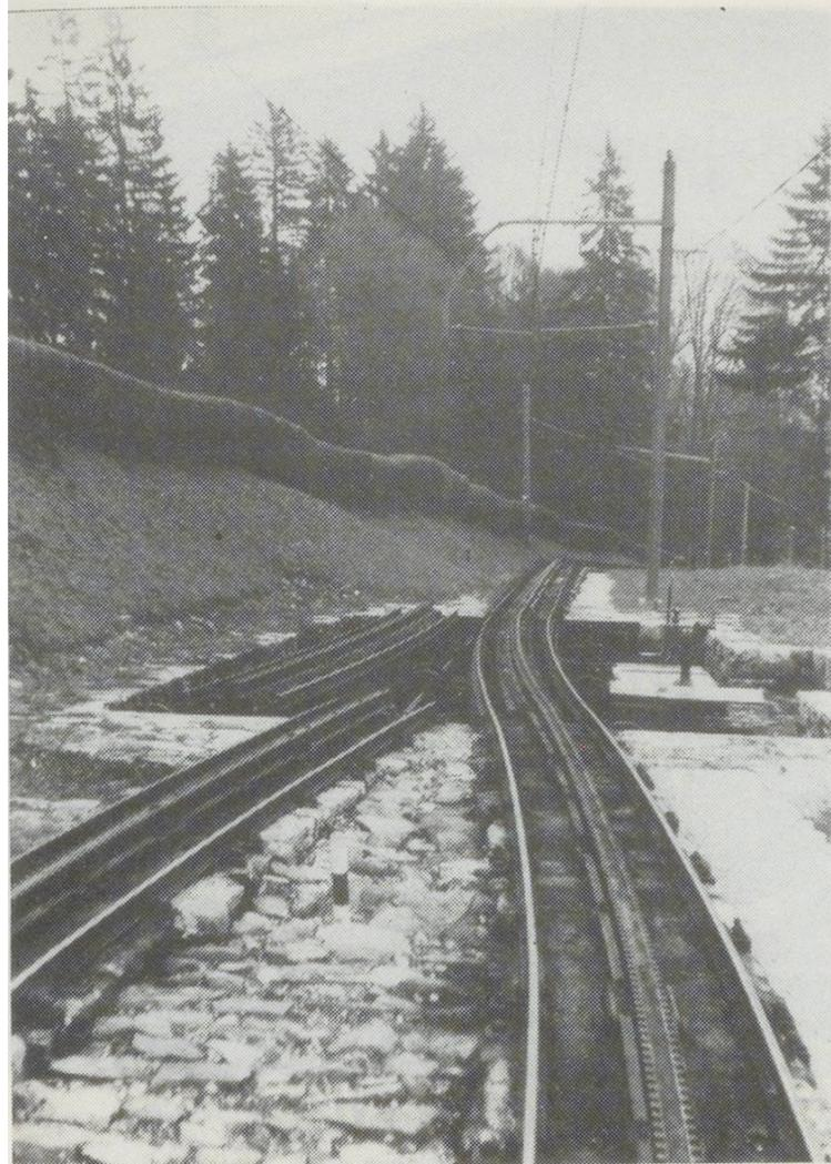
Traverser "points" at Aemsigenalp passing loop.
