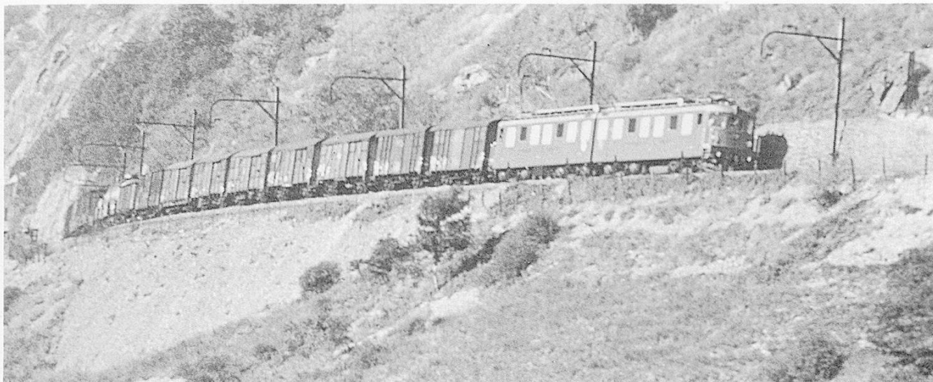
Freights in 1967 were mostly composed of short-wheelbase wagons, as is this example behind a BLS Ae8/8, a short distance from Brig
