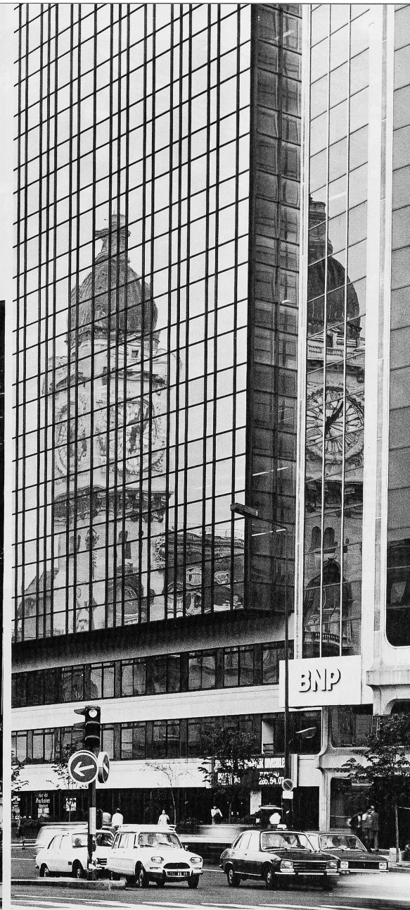
The Gare de Lyon, one of the six great railway terminals in Paris, was built around 1900. The clock-tower, characteristic of the railway architecture of the 19 th century, had a symbolic meaning in addition to its practical function and competed with the old city landmarks, such as church steeples and town gates. Today it is reflected in the glass fronts of high-rise buildings that hem it in
