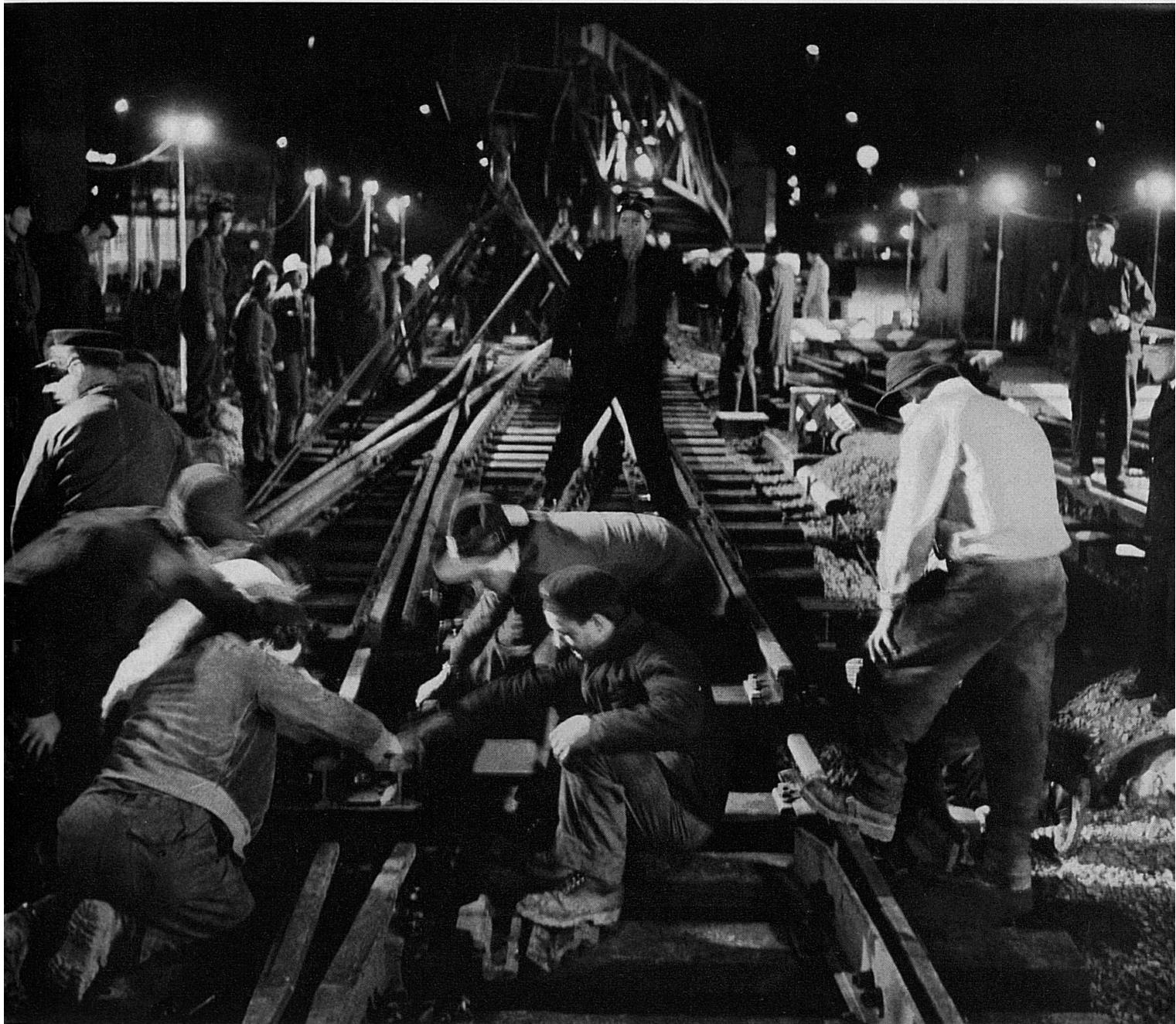
*After old switch units are removed, cranes lower the new units into position (above). Final details, of course, (left) have to be handled manually by skilled track crews.*
