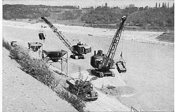
Draglines, 90 tonnes, 1 m³.
