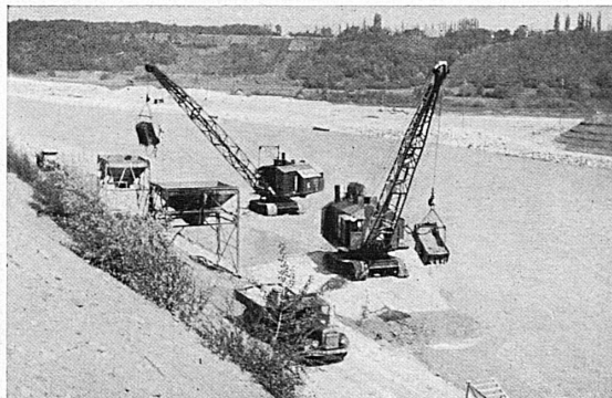
Draglines, 90 tonnes, 1 m³.
