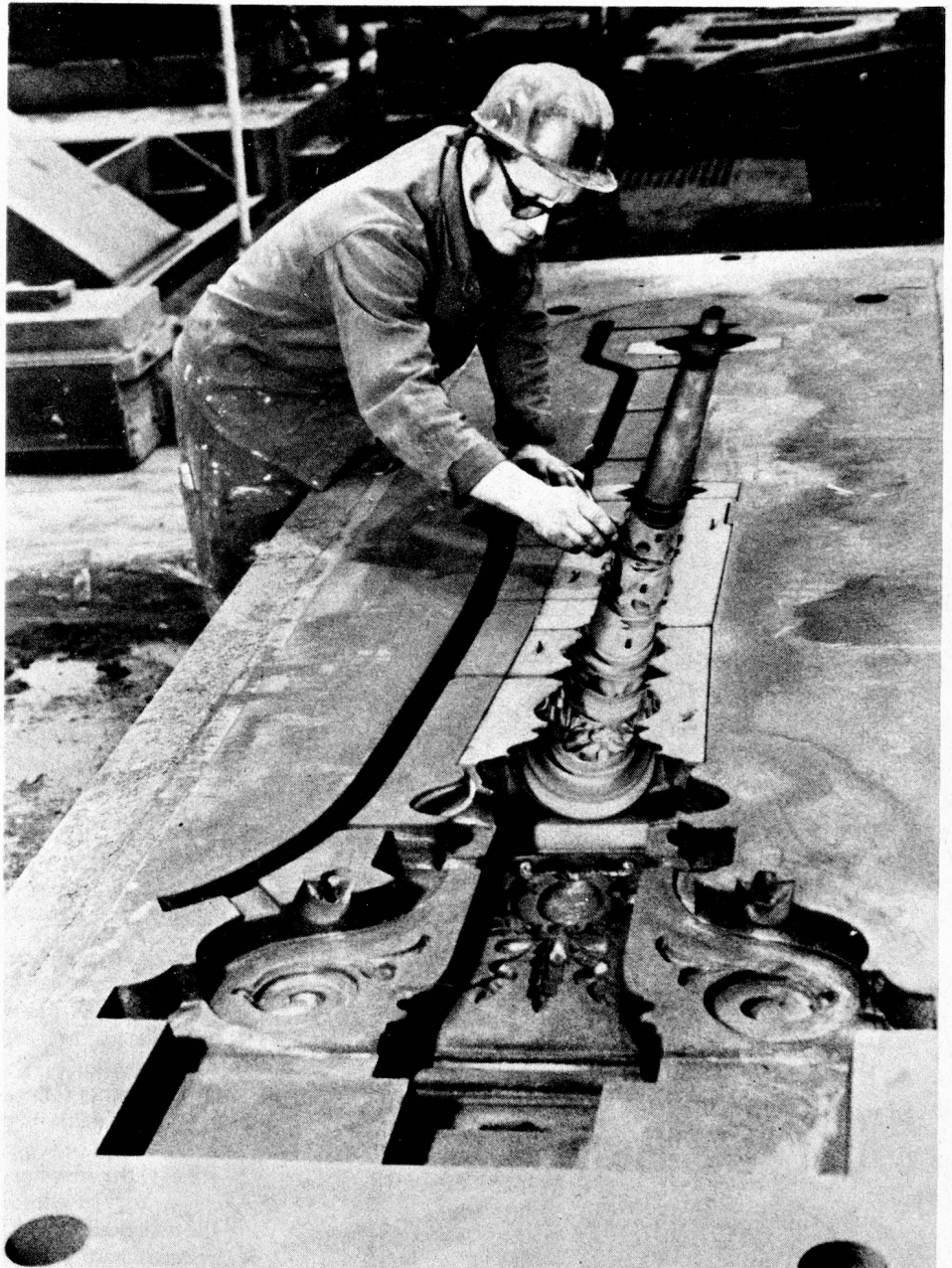
Fabrication in Sulzer foundries of the casting pattern for the lamp-posts for the Munter bridge in Zürich. See photograph on front cover.
