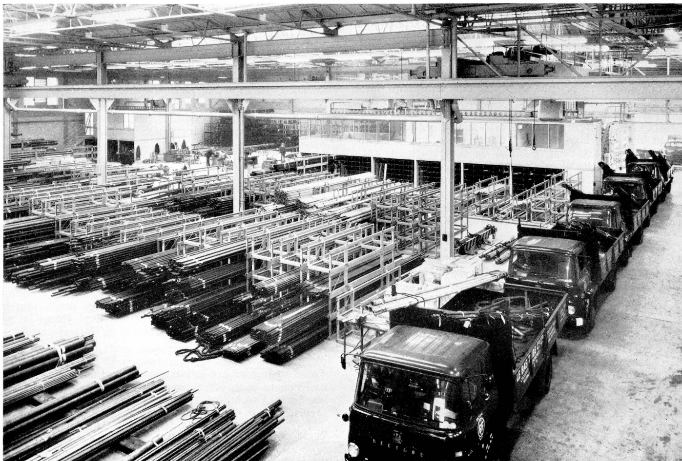
General view of the steel tube warehouse and loading bay at the new Le Bas London Distribution Centre.
