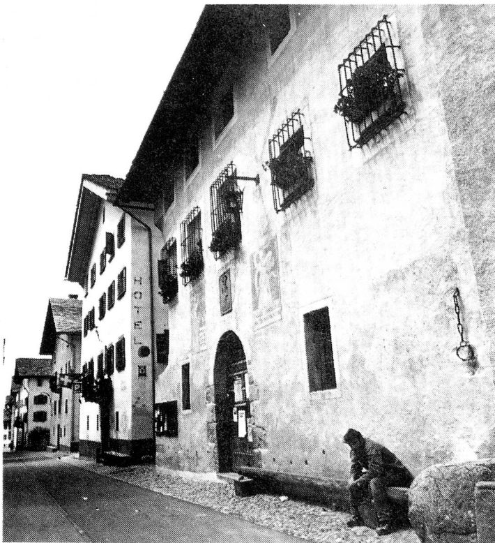
The Commune Hall of Vicosoprano. Note the neck fetters on the wall
