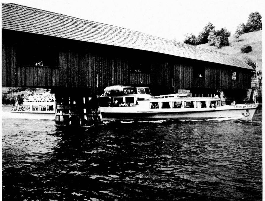
Covered wooden bridge going over the river Rhine
