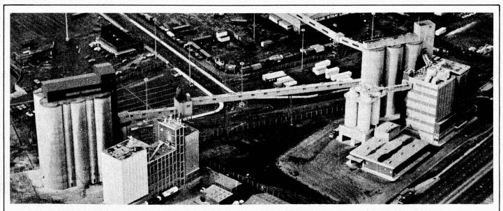
The new harbour in Seaforth, Liverpool. On the left in the foreground is Allied Mills Ltd. flour mill, 280 t/24 hours, with grain silo 17000 tons. On the right is Kellogg Co. of Great Britain, 720 t/24 hours corn mill, with 7500 t silo. Both mills were built by Bühler Brothers in 1972/73.
