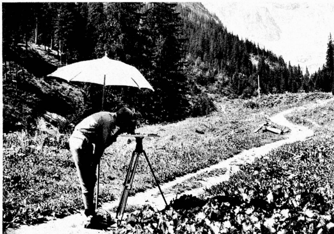
Topographical details were surveyed using the planetable
