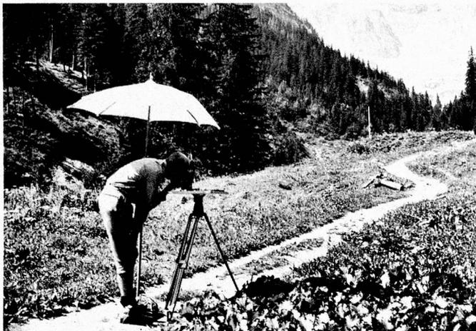
Topographical details were surveyed using the planetable
