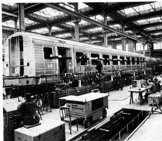
Erection of a CFF wagon at Neuhausen (SIG).
