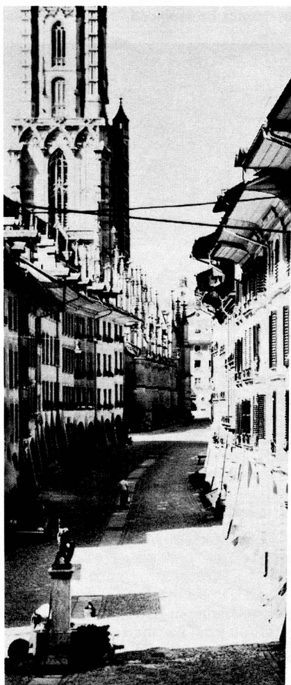
The Junkergasse, one of Berne's old streets
