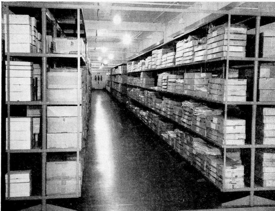
The illustration shows Acrow Cantilever Shelving installed in the Guildford branch stockroom of Marks & Spence Ltd.
