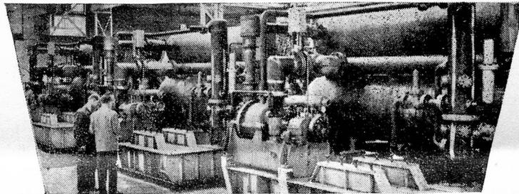
Two plants produce 700 tons of refrigeration for 'Tower Block' with another 450 tons capacity plant in 'Y Block'.
