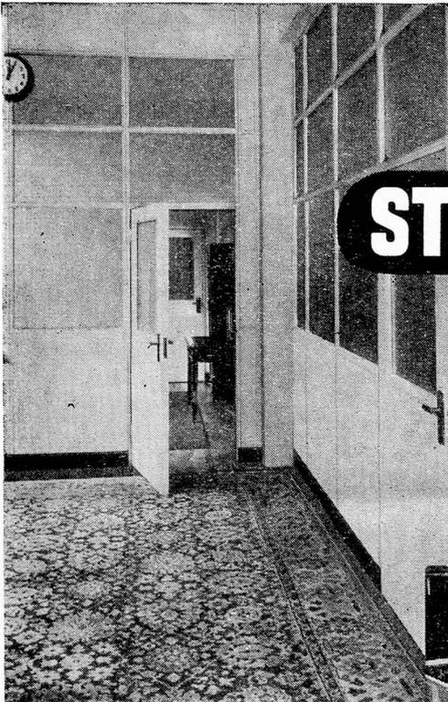
They can be dismantled and re-erected to suit any change of plan
