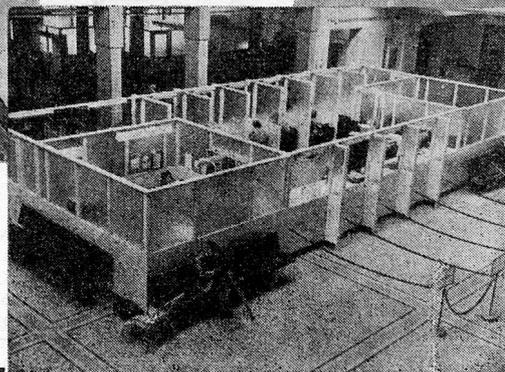
**They can be dismantled and re-erected to suit any change of plan**
