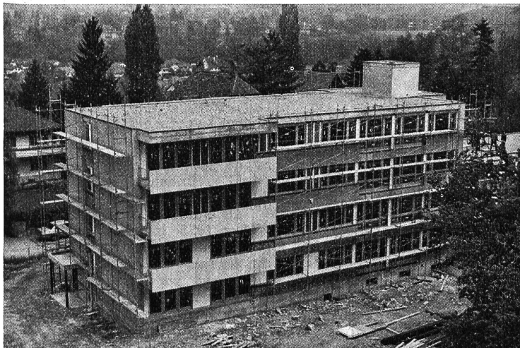
Neubau in Wabern
