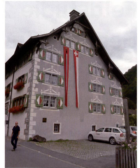
Suworow-Haus in Elm.
