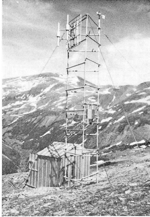
Figure 2 Station basse. Pylône et refuge
