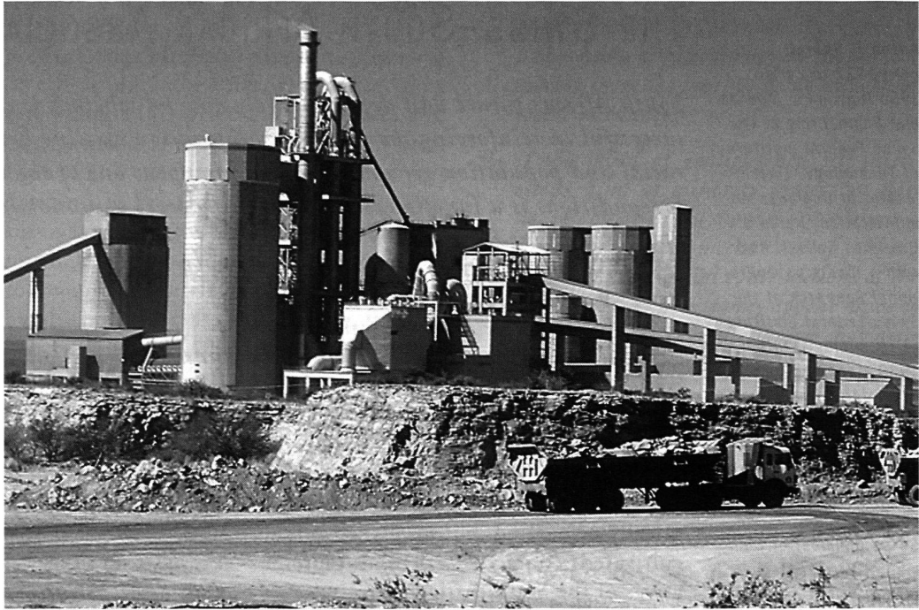
The Ulco cement factory in Kimberley, which belongs to Alpha Ltd., a South African subsidiary of Holderbank.
