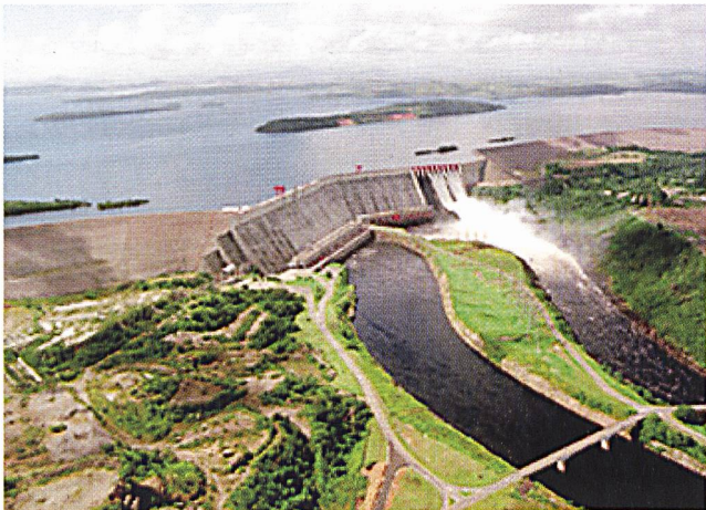
The Guri Dam is the world's second largest hydroelectric plant in terms of power production capability. It has two powerhouses, each containing ten hydroelectric generating units; the total capacity of the 20 generating units is 10 000 MW (photo Edelca).
