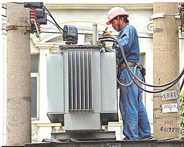
Montage eines Transformators in Shanghai.
