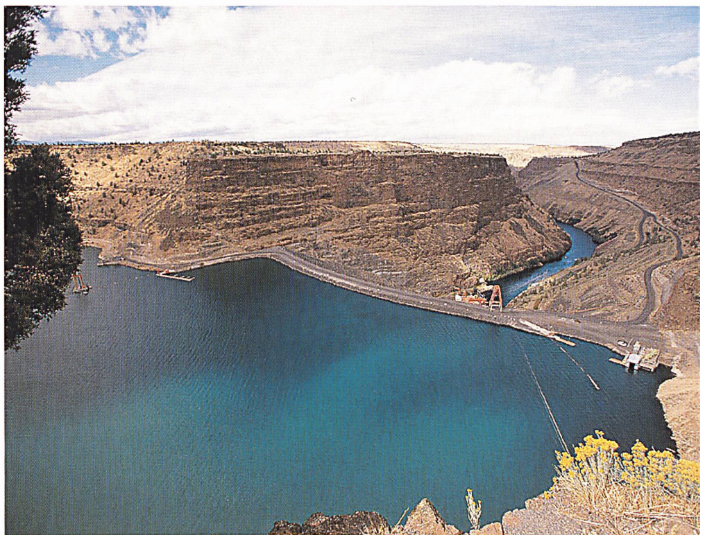
Lake Billy Chinook at Round Butte Dam (photos: Portland General Electric/PGE).
