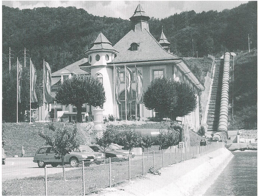
Figure 2 ELECTROBROC: un site remarquable
