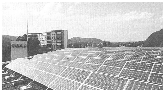
18-kWp-PV-Anlage in Liestal (Flachdachmontage)
