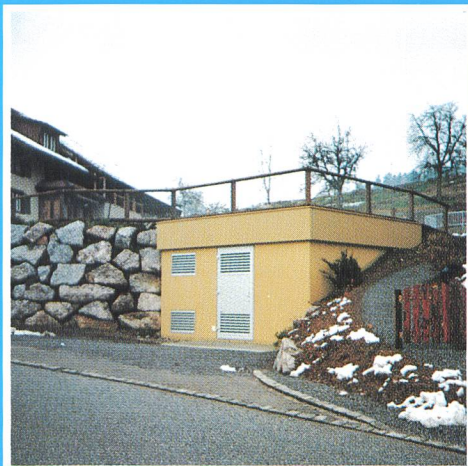
Station en talus Hangeinbaustation in Gossau/ZH
