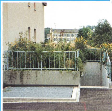
Station souterraine Unterflurstation in Sisseln/AG
