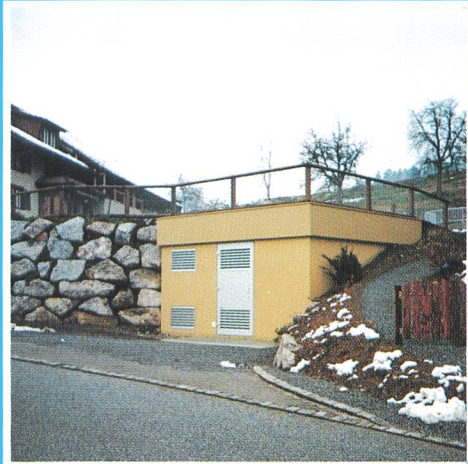
Station en talus Hangeinbaustation in Gossau/ZH
