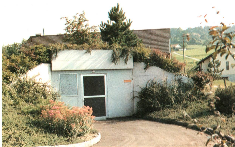
Hangeinbau-Trafostation EW Gossau
