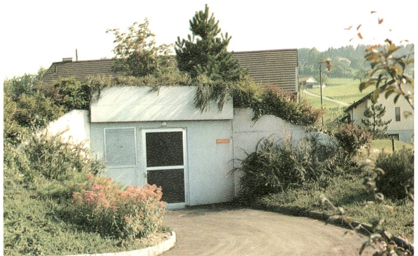
Hangeinbau-Trafostation EW Gossau
