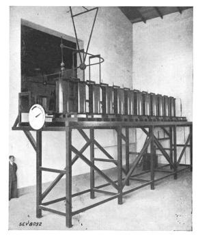
${\rm Fig.~1.} \\ 12 {\rm stufiger~Stossgenerator~f\"{u}r~Spannungen~bis~1200~kV}.$
