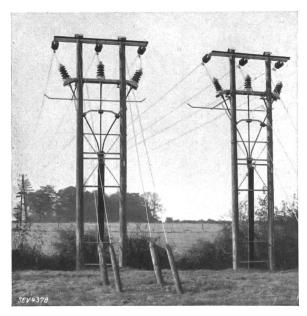
Fig. 11. «Rural Electrification». Kabelendmasten 33 kV. (Photo Henley.)
