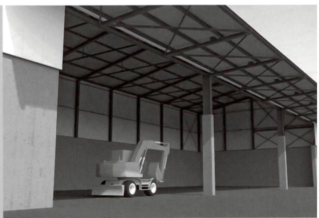
as snow can be moved by the wind and slide from the roof onto the canopy below. The snow and wind loads are carried by the girders, which are designed as trussed beams. Special attention was paid to the use of compact components and simple assembly.
