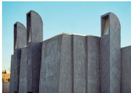
01 Islamic Center Albuquerque (1985-86). Architektur: Bart Prince, Albuquerque (Foto: Bart Prince)
