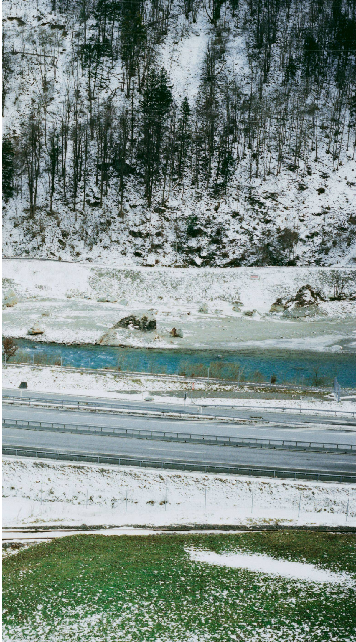
07 Complete renovation of the highway through Uri Valley (photo: Jules Spinatsch)
